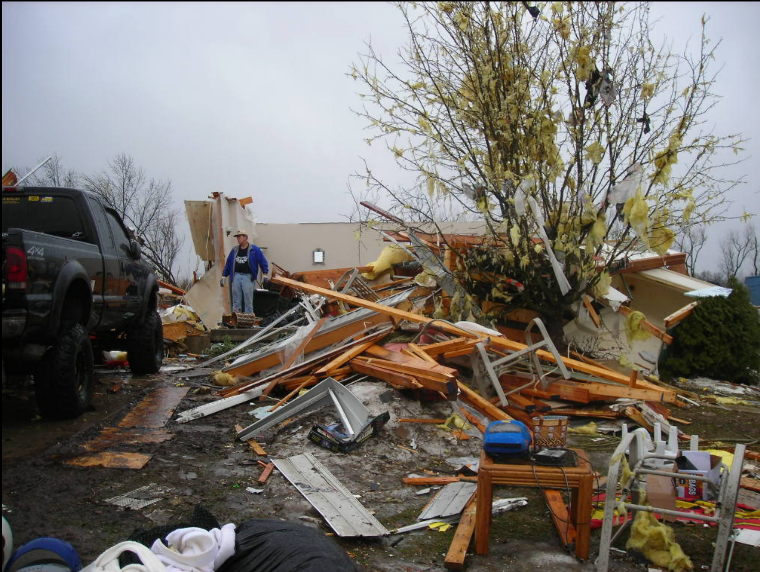
The front of what is left of the house from the driveway. Note the insulation in the tree.
