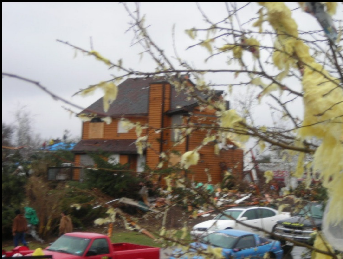
The neighbor's house to the NE
