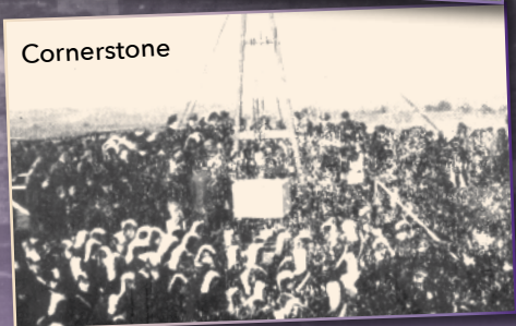
Sherman Hall Construction
