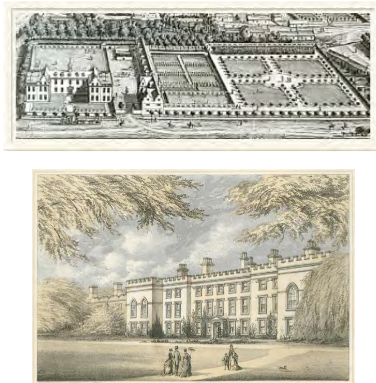
Figure 1.2: Views of Kirkleatham Hall before and after remodelling in 1763.
